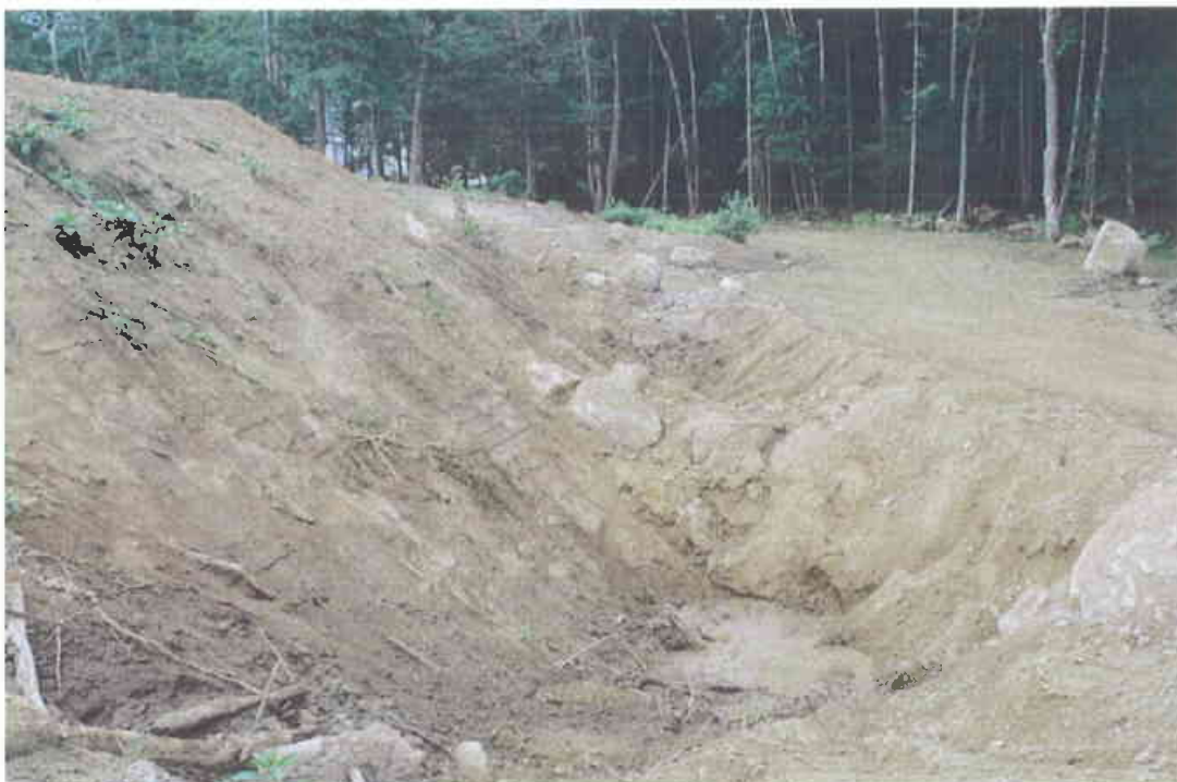
Photo 3C Maintained interim sediment basin traps on NC/HF property. View looking to the east.
