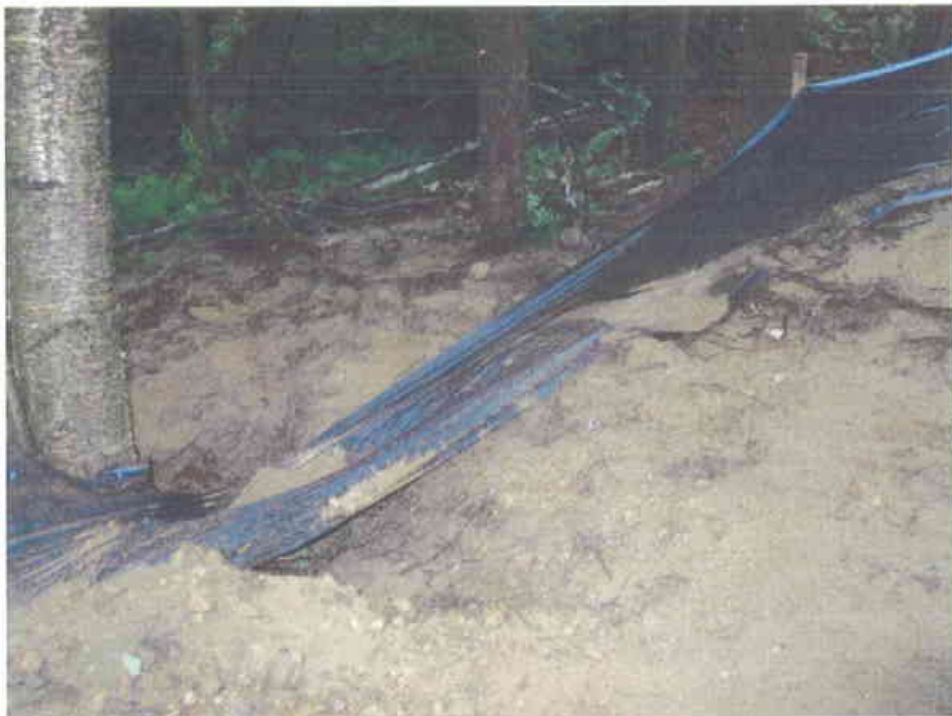
Photo 14 B Silt fence undermining on NC/HF access drive.
