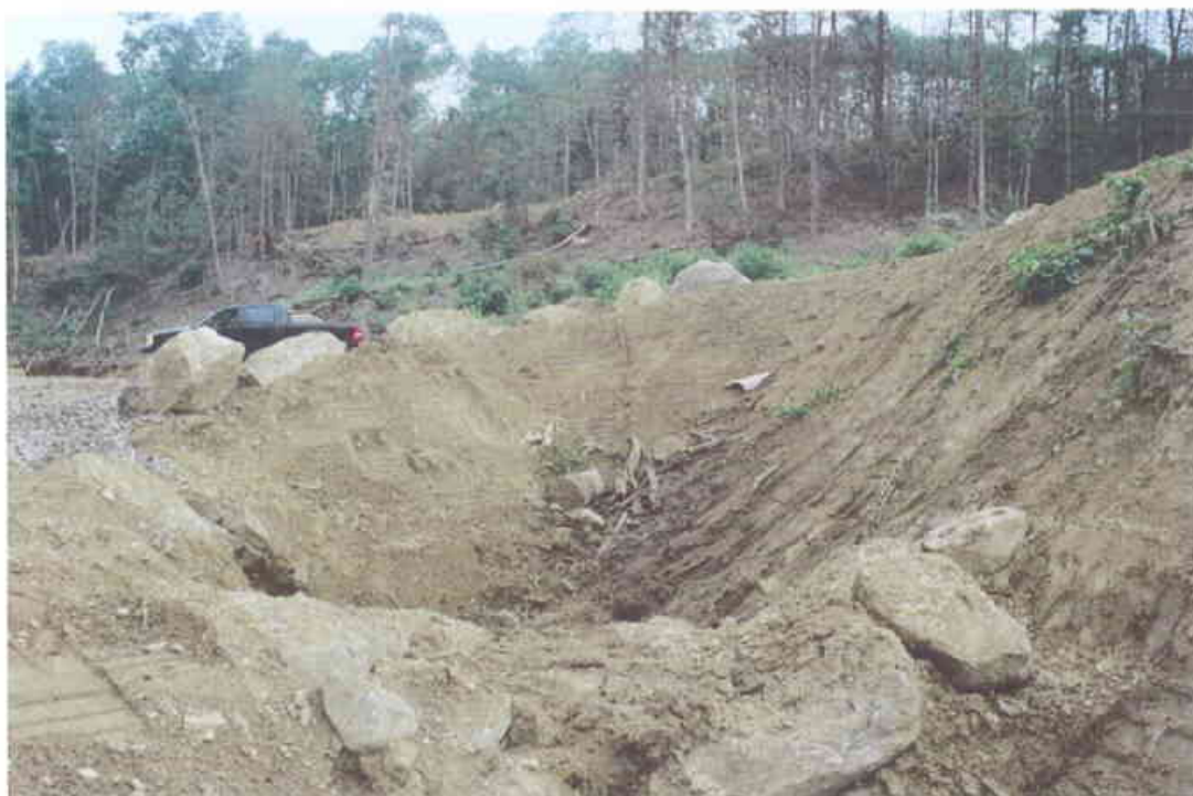
Photo 4C Maintained interim sediment basin traps on NC/HF property. View looking to the west.
